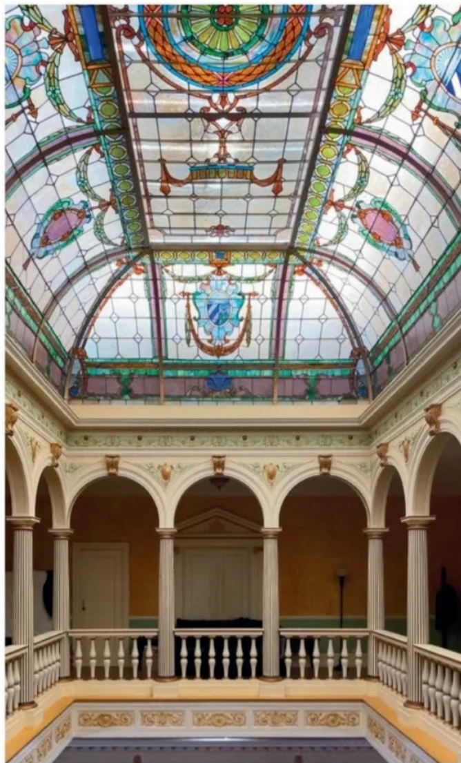
Above left, at the Cuban Embassy in Washington, D.C., Lynchburg Stained Glass removed the 1917 building's stained-glass skylight that crowns its four-story atrium, preserved it, re-leaded it, and reinstalled it. Right, Lynchburg Stained Glass removed, restored, and preserved eight historic stained-glass windows at the Chapel of the Centurion at the Fort Monroe National Monument in Hampton, Virginia.
